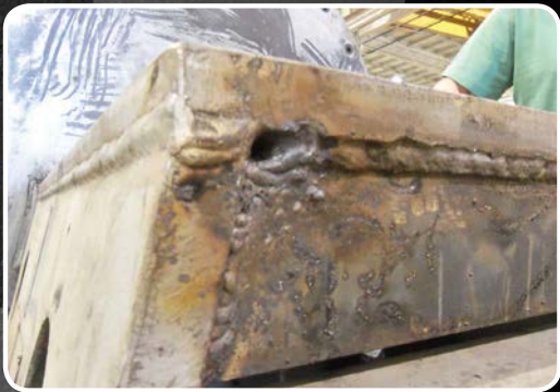
Poor welds and construction of the existing fan caused excess vibration
