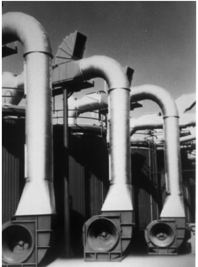
Figure 6. Well-designed duct configuration
