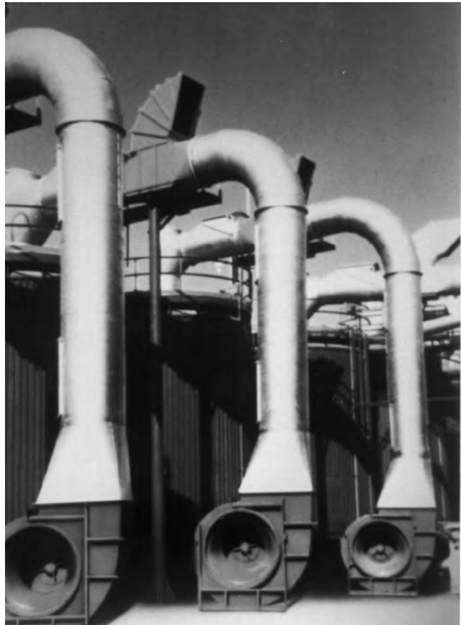
Figure 6. Well-designed duct configuration
